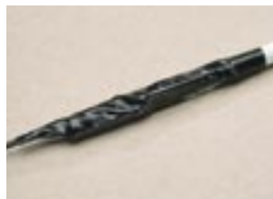
Attaching a wire to a fish tape: Strip the jacket off the cable. Bend the conductors over the fish hook. Wrap the fish and the cable with electrical tape.
