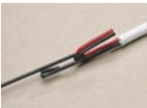
Attaching a wire to a fish tape: Strip the jacket off the cable. Bend the conductors over the fish hook. Wrap the fish and the cable with electrical tape.
