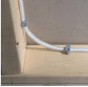
No sharp bends: When you turn a corner, use a gradual bend. Sharp bends can damage the wire.
