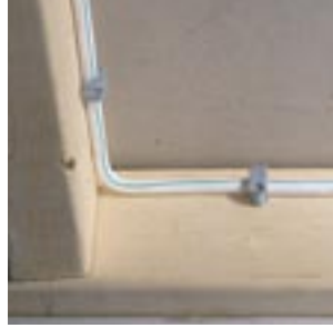
No sharp bends: When you turn a corner, use a gradual bend. Sharp bends can damage the wire.
