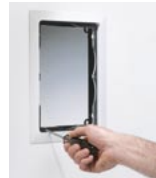
D. Attach outer frame to bracket placed behind the wall.
