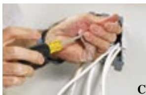
Installing wall plates for speakers: A. Insert the wires into the J-box
