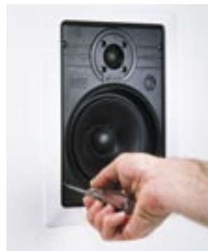
E. Connect the wires and screw the speaker into the frame.
