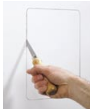
C. Cut the drywall out in one piece.
